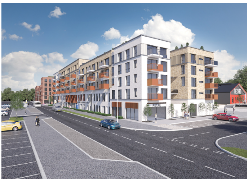
Block H - Street View - Havannah Way
